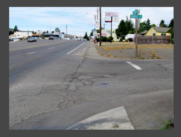
In addition to replacing ADA curb ramps, ODOT will also pave crosswalks and side street approaches, like this one at Baker Street, that are damaged or heavily cracked.
