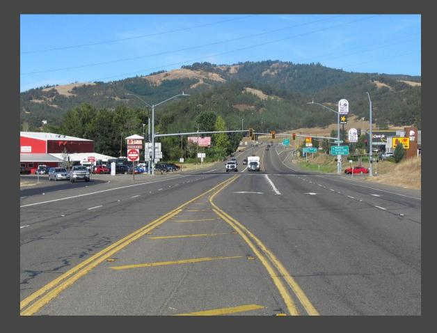
At the Grant Smith Road intersection, **ODOT** will install raised traffic separators and concrete islands along the center median, adjust the roadway to better accommodate Uturns, and upgrade sidewalk curb ramps.
